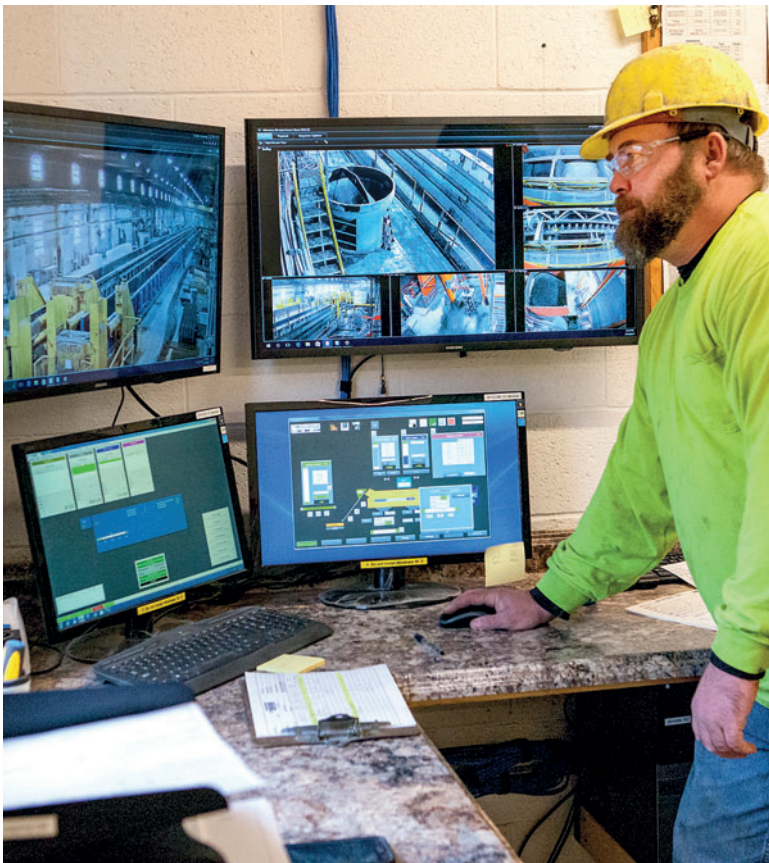
Figure 13: NPP plant operator John Shala mans the PC-based control system for the NPP's new ACT/Wiggert MobilMat Mo4500-5-WCS batching system.
