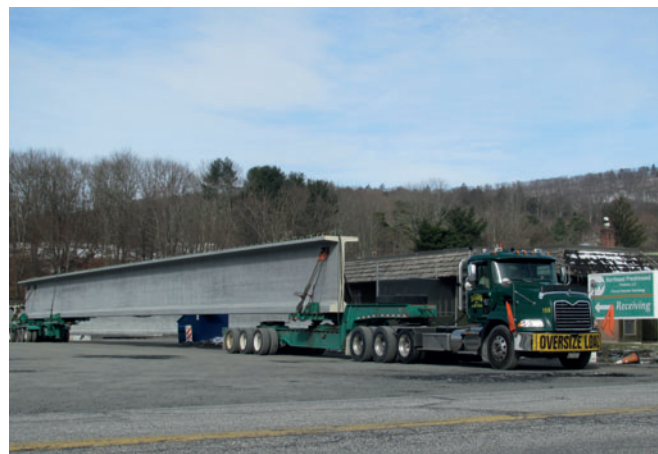
Figure 4: Northeast Prestressed Products is providing 400 precast, prestressed concrete bulb-T beams to the US$1.5 billion Goethals Bridge Replacement Project. Here, a 178-foot long, 110-ton bulb-T is loaded on a truck equipped with steerable trailers that enable the rig to negotiate sharp turns.
