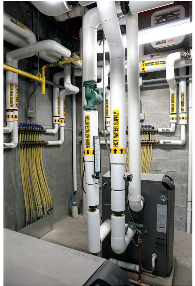
Figure 8: ACT engineers worked closely with NPP and mechanical contractors James Craft & Son, Inc., of Manchester, Pennsylvania, to help specify and design the new aggregate storage system. The five-compartment aggregate storage system is equipped with radiant heating capable of maintaining fine and coarse aggregates at approximately 65-75°F.
