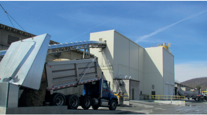
Figure 6: New batch plant at Northeast Prestressed Products in Cressona, Pennsylvania, USA, is fully enclosed to provide all-season consistency.
