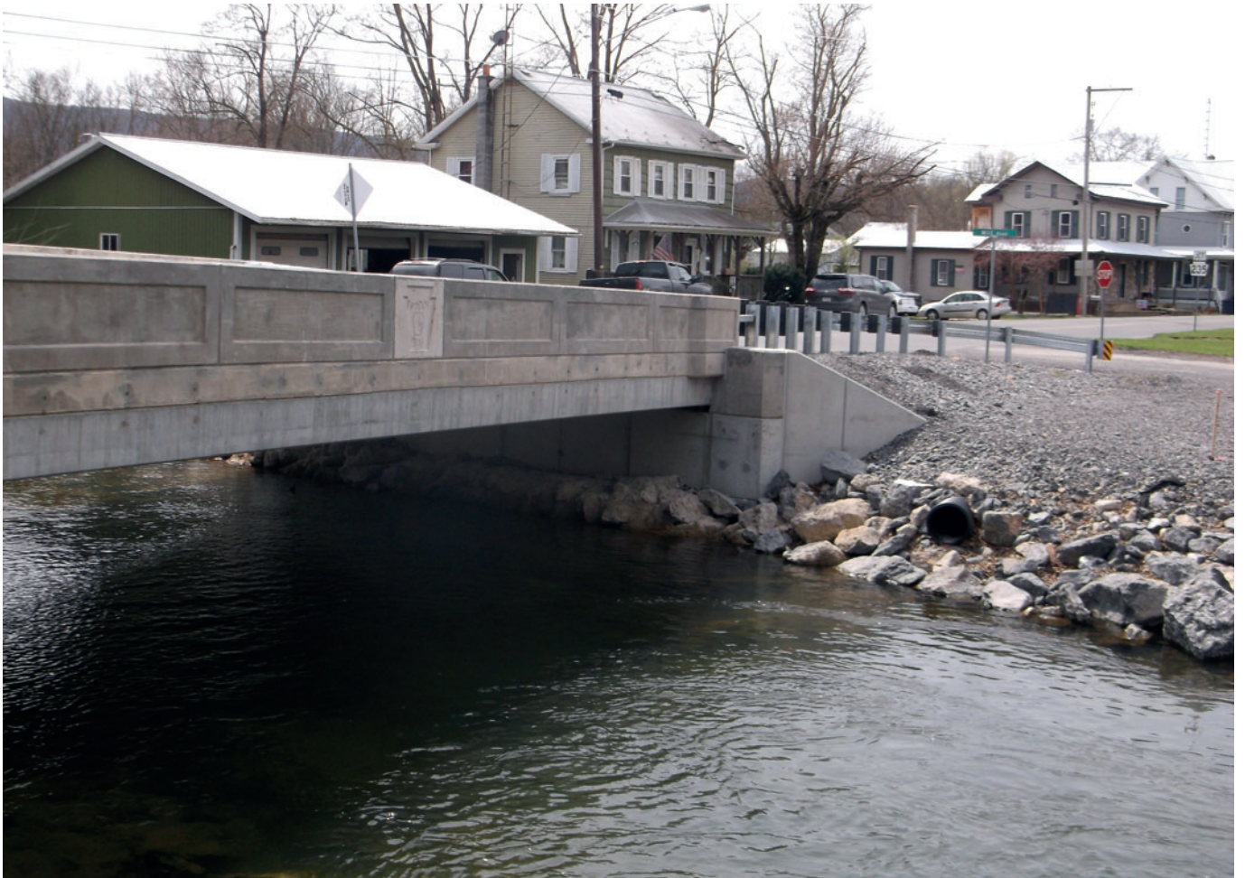
Bridge 184 after replacement
